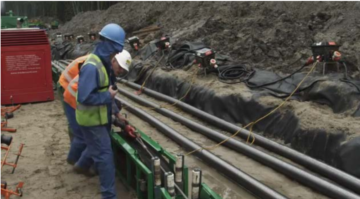
Figure 2: Laying roadside underground cables in conduit
