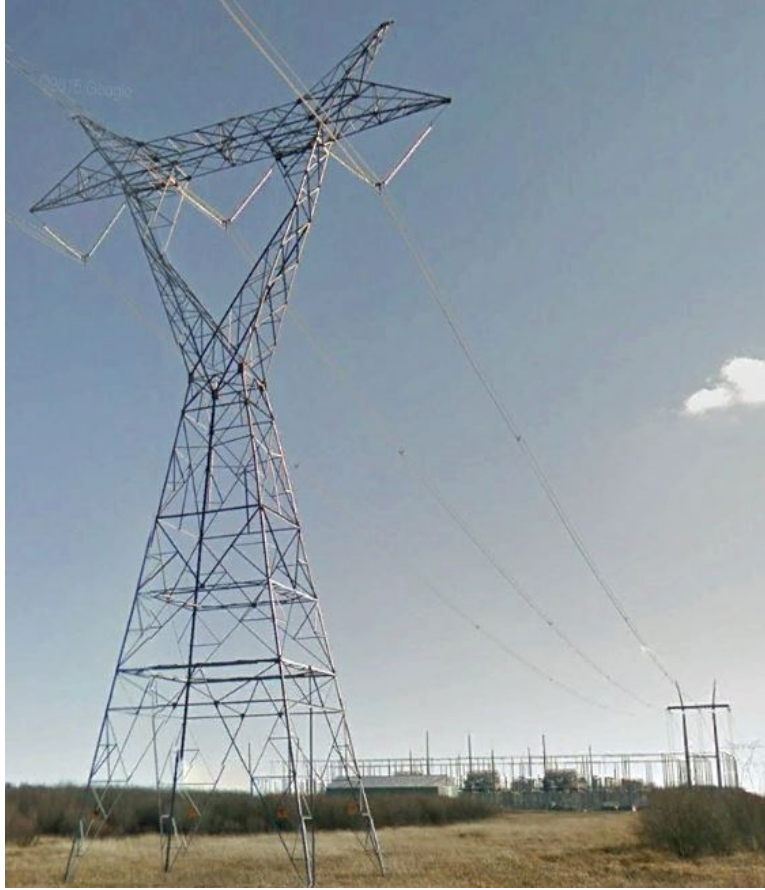
Figure 8: The series capacitor station for the existing M602F transmission line near Warroad, Minnesota (Google Earth)
