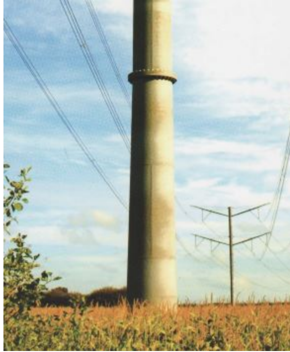
Figure 3: New double circuit tubular 400 kV AC transmission line in Denmark 1 [1]
