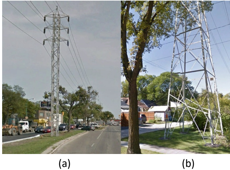
Figure 13: Transmission structures on Pembina Hwy (a) and Grant Ave (b) that might cause property damage with structure failure (Google Earth)
