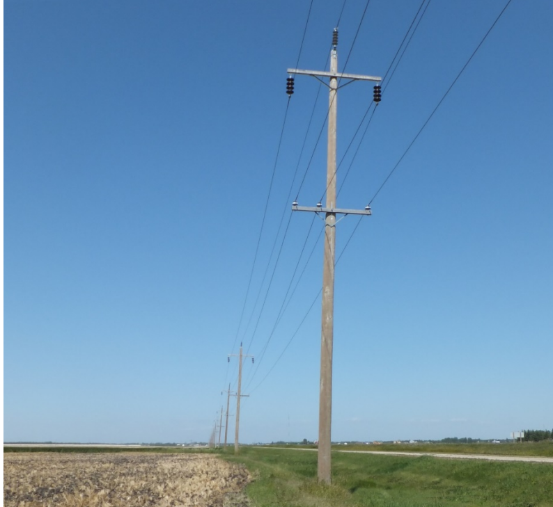
Figure 16: Typical rural roadside 66kV feeder
