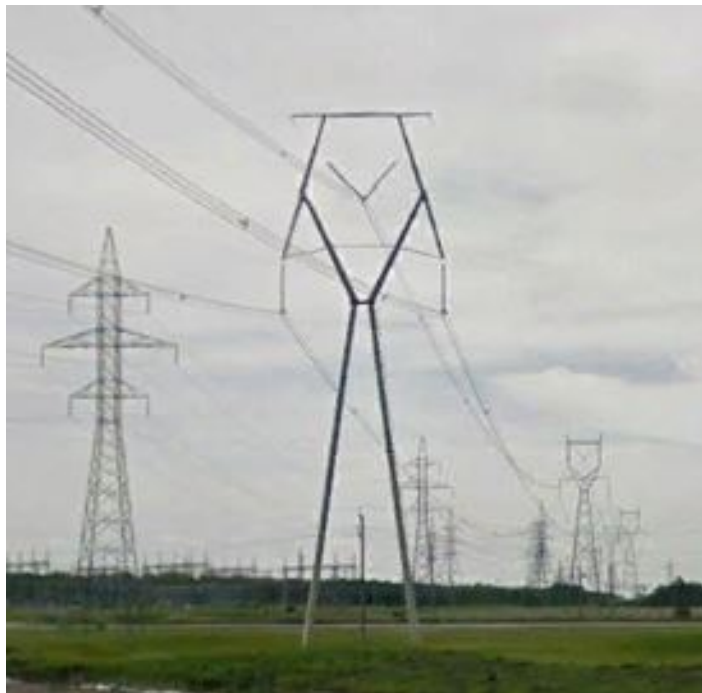
Figure 5: A single Manitoba Hydro tubular steel aesthetically designed 500 kV transmission tower but which is not low profile (Google Earth)
